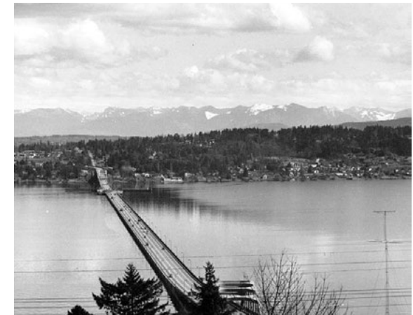
Lake Washington Floating Bridge, n.d. Unknown Photographer, Courtesy University Libraries: University of Washington Special Collections & Museum of History & Industry (MOHAI). Image Number: SEA0936
